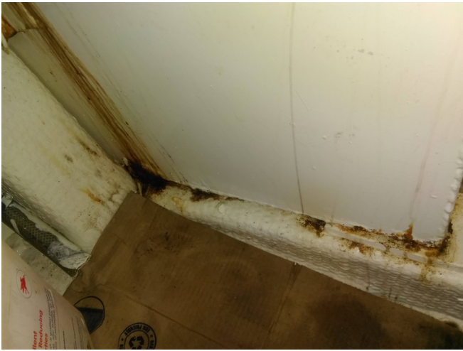
Figura 2: left tank rusty
