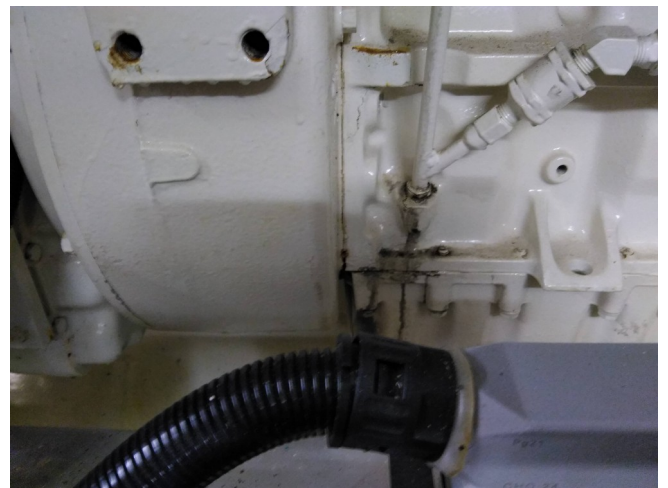
Figura 3: left engine leak
